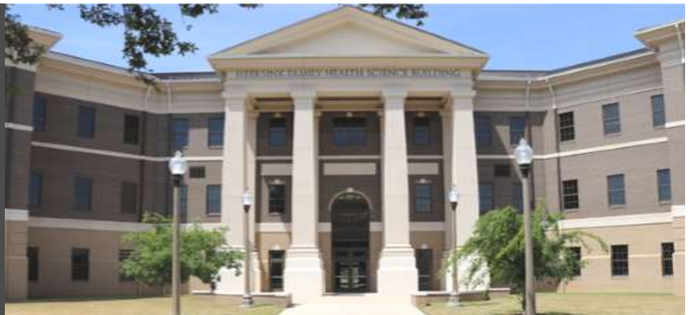
Heersink Family Health Science Building
