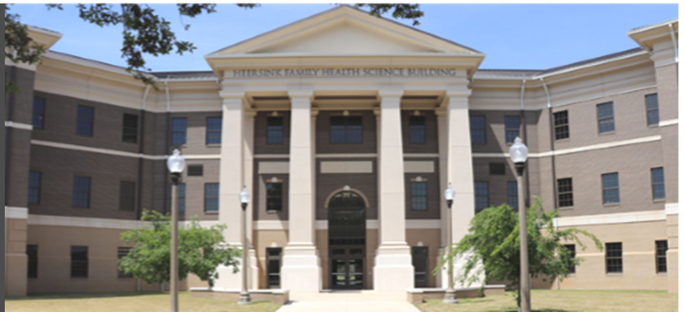
Heersink Family Health Science Building
