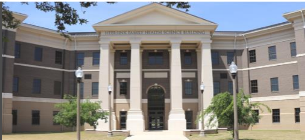
Heersink Family Health Science Building
